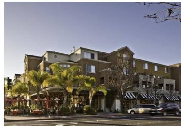
City Center Plaza - Redwood City
